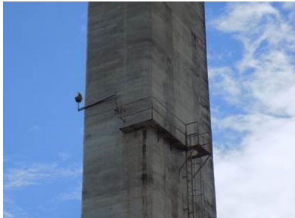
Figure 9 - Lack of maintenance and absence of signalling equipment. Source: collection of authors (2016).
