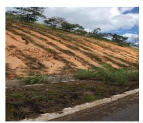
Figure 5 - Laminar erosion on a slope at point P10 along the TO-445 road. Source: author (2019).
