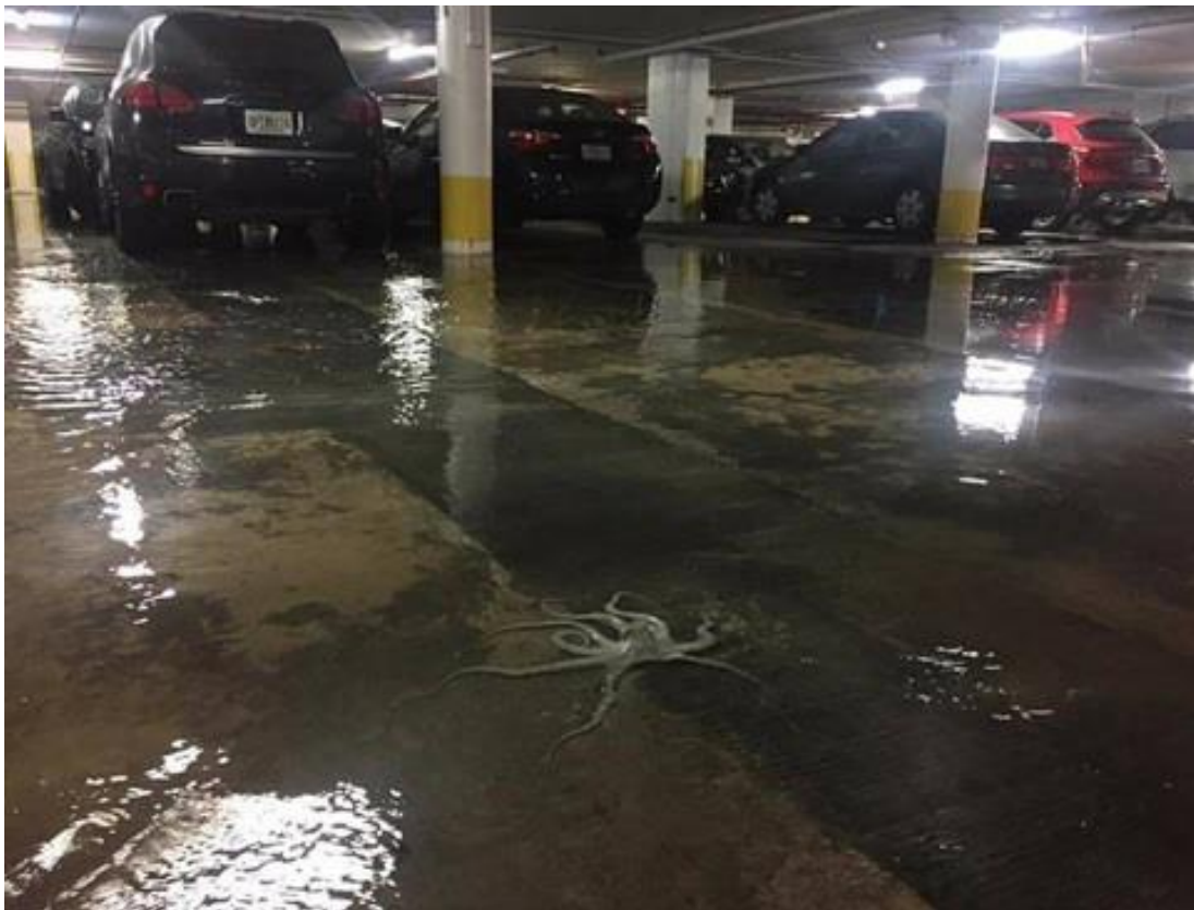
Figurea 5 – Presence of marine fauna in coastal building parking lots in Miami. Source: Richard Conlin for Miami Herald Newspaper (2013).
