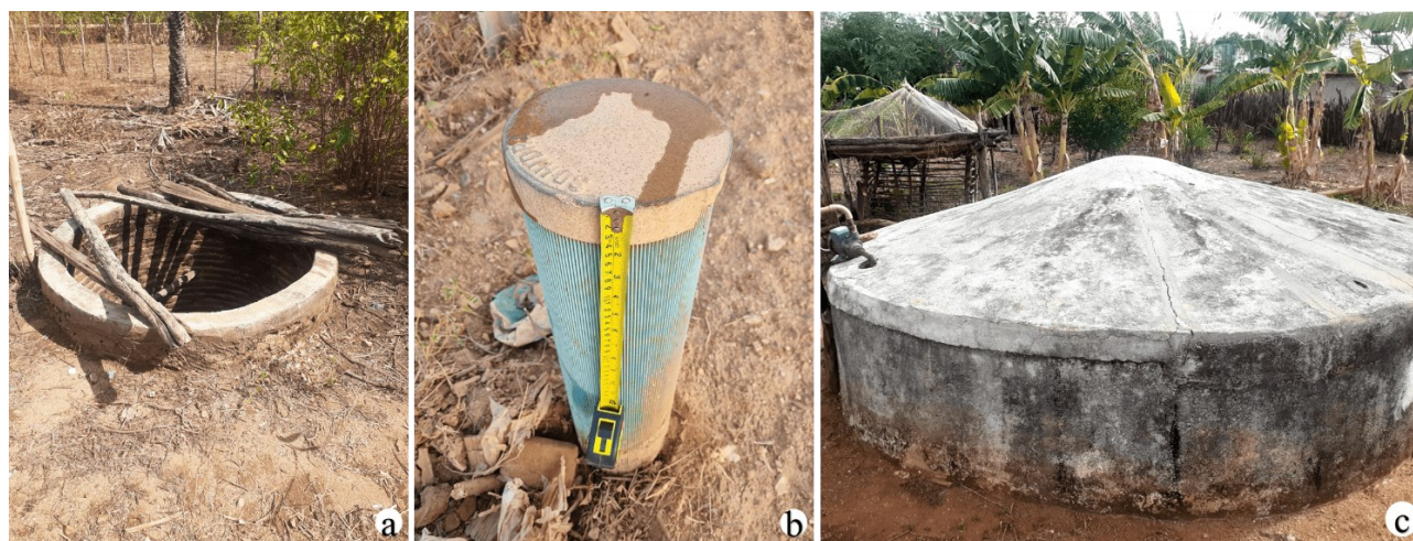
Figure 3 – a - Amazon well; b - tubular well; c – plate cistern, in the lower course of the Groaíras River, Ceará. Source: Authors (2025).
