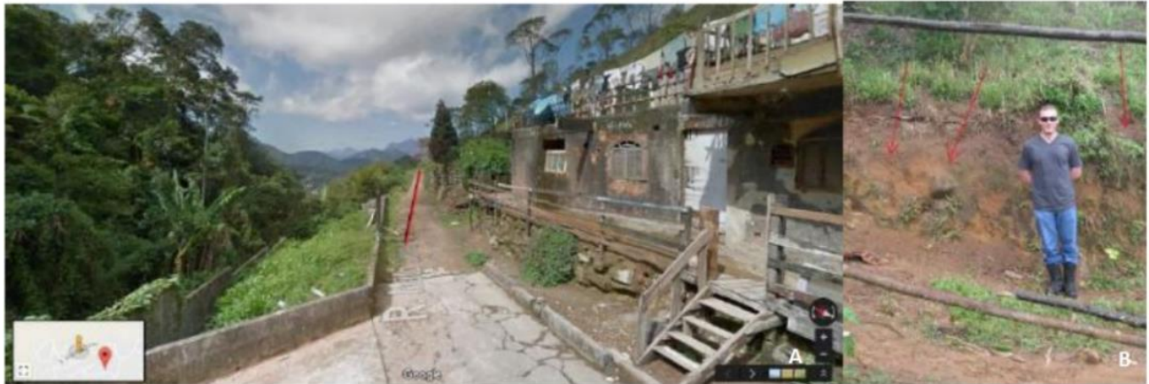
Figure 3 - (A) Location of line 1 data acquisition. (B) Reddish soil coloration of the soil. Source: Marques (2016).
