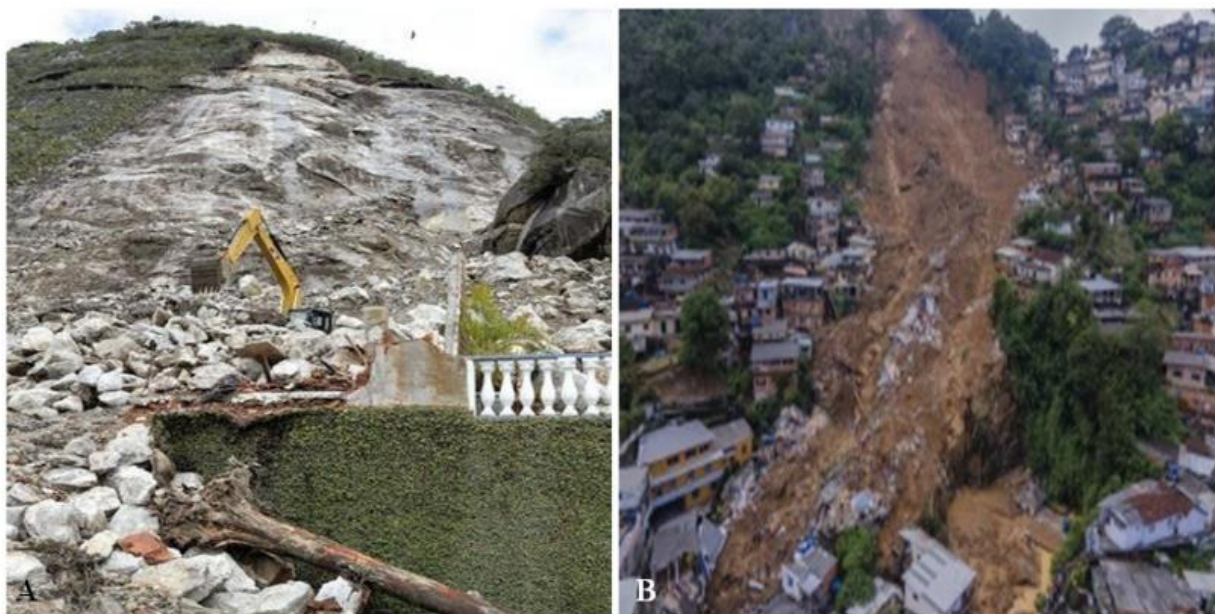
Figure 15 - (A) Block falls recorded in the Quitandinha neighborhood in 2017. Source: G1 (2017). (B) Race on Morro da Oficina (Petrópolis) Source: Folhapress (2022).
