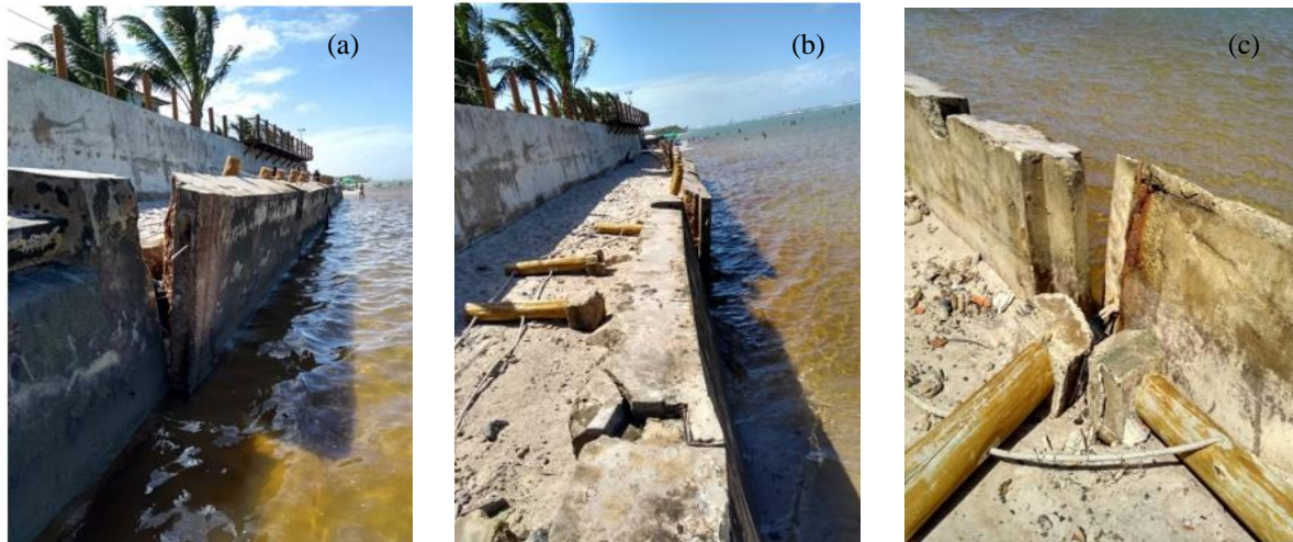
Figure 4 – (a,b,c) situation of the existing maritime retaining wall, Ipojuca/PE. Source: Authors (2023).
