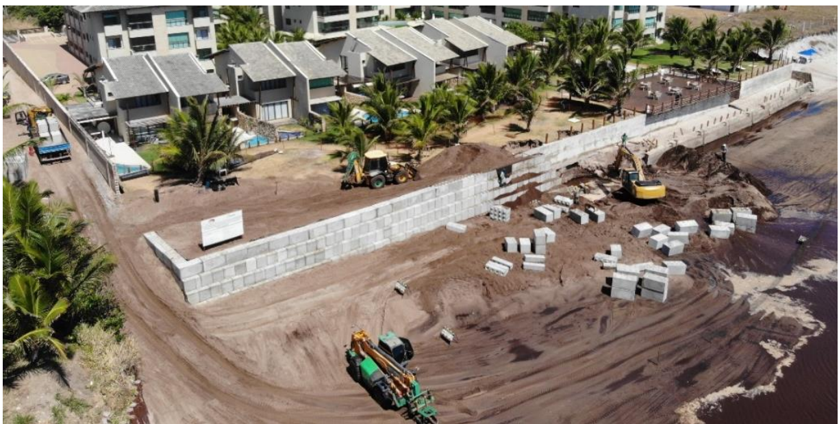
Figure 12 – Maritime containment execution / Ipojuca -PE Source: Authors (2019).
