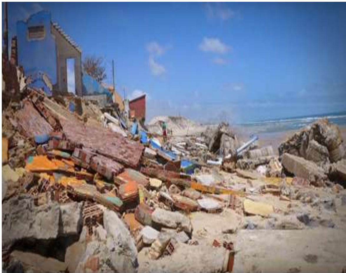
Figure 7 – Debris at the seaside of commercial structures on Morro Branco beach destroyed by the sea. Source: Eduard Sweets, 2016.
