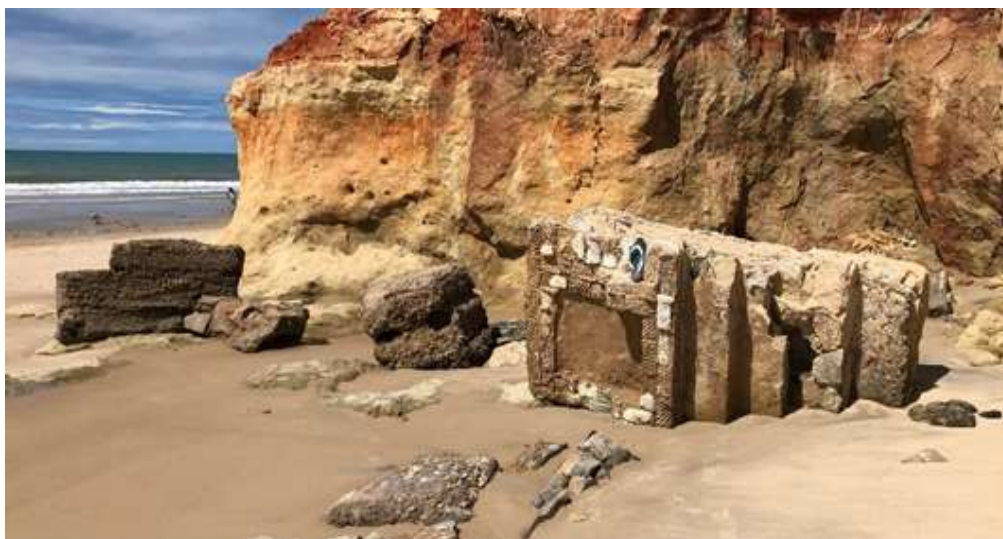
Figure 5 – Debris from summer residences located on the Morro Branco beach strip. Source: Prepared by the authors.
