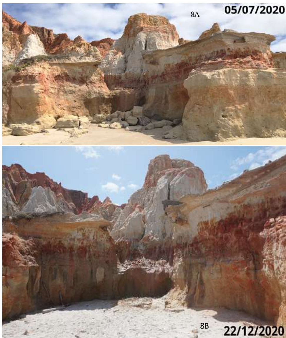
Figure (8) (a) and (b) – Sample of the removal of coarse material provided by the mass movement. Source: Prepared by the authors.
