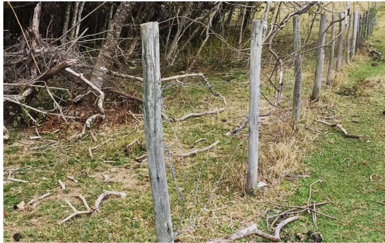
Figure 9 – Fence in a poor state (notice the broken wires) at spring 8. Source: Prepared by authors (2022).
