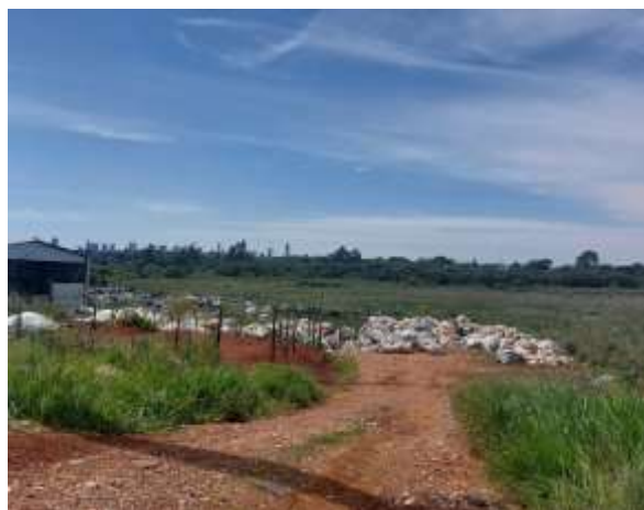
Figure 6 – Area for storing recycled material. Photo: Fabiula Eurich Machado (2023).
