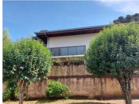
Figure 8 – Two-storey masonry house. Photo: Fabiula Eurich Machado (2023).
