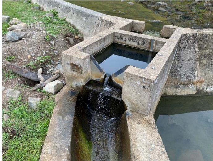
*Figure 9 – Triangular Flow Meter.
