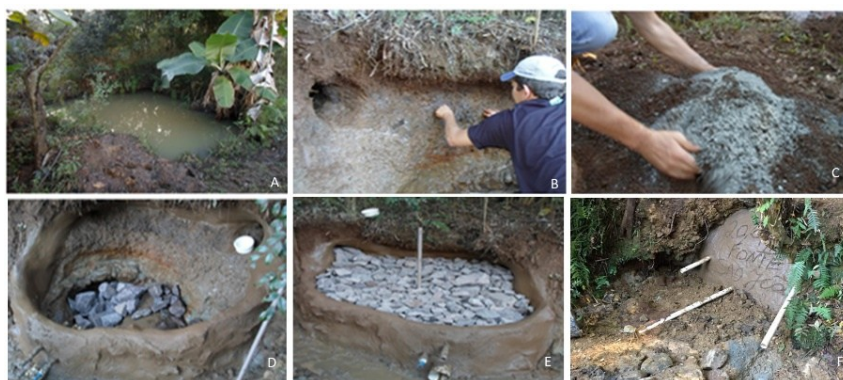
Figure 1 – Recovery of the spring through the soil-cement method. A) Spring is to be recovered. B) Spring cleaning. C) Mixture of soil and cement. D) Construction of the mini dam. E) Spring being covered by rock fragments. F) A recovered and functioning spring.
