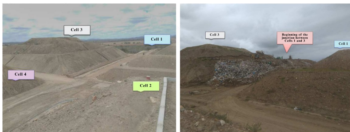
Figure 2 – Landfill cells: (a) prior to the initiation of the joining process and (b) following the commencement of the joining process.
