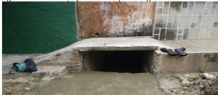
Figure 1 – Excessively open manhole producing a hazardous situation.
