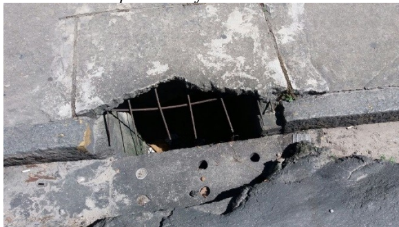
Figure 4 – Damaged manhole cover with exposed reinforcement bars: serious risks for pedestrians or cyclists.
