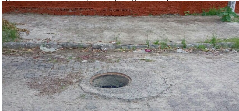
Figure 5 – Manhole missing cover, posing a risk to pedestrians or vehicles.
