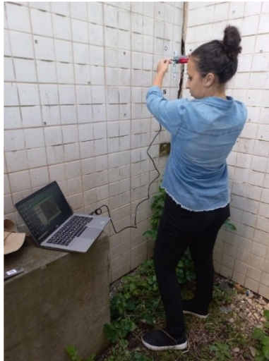
Figure 2 – Structured light scanning of the crack. Source: The authors (2026).
